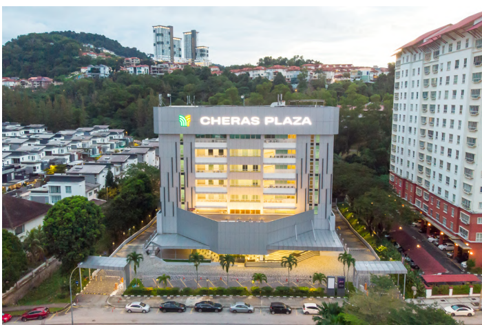
Efforts at Cheras Plaza are focused on achieving and maintaining a 3-star rating under the Energy Commission’s Guidelines
