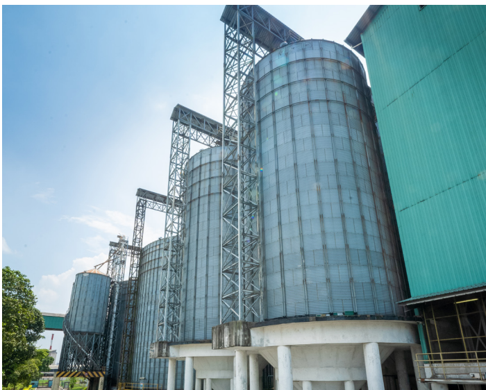
FFM's flour and feed mill silos in Pulau Indah, Selangor
