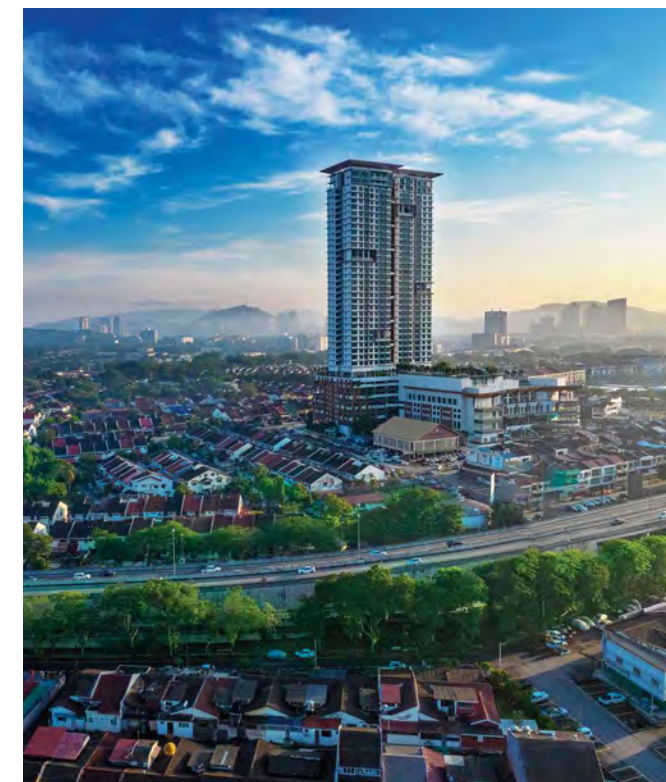
PPB Properties' latest development, Megah Rise in Taman Megah, Petaling Jaya
