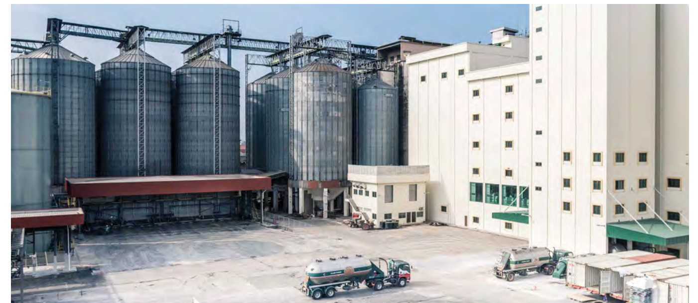
Flour mill complex and wheat silos in FFM Grains & Mills, Pasir Gudang
