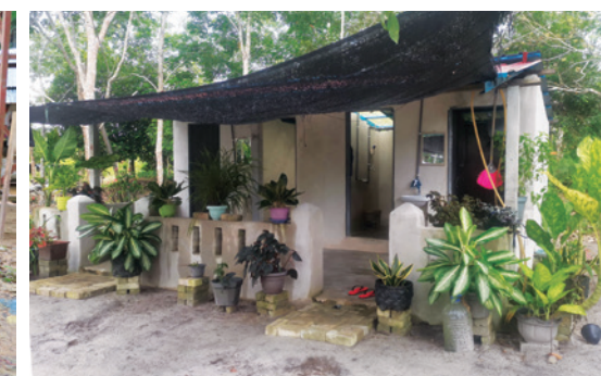
Community sanitation facility contributed by the Group
